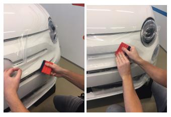
For curved areas, it is necessary to firmly pull and stretch the film in order to conform the film around the surfaces. It is recommended to stretch the material without applying any heat, making use of the intrinsic flexibility of the film. It is also possible to gently heat the material to a
